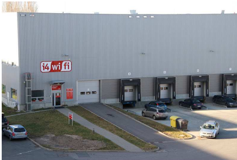
3800 m2 of storage area
