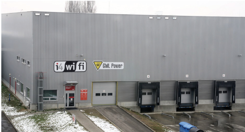
3800 m 2 of storage area
